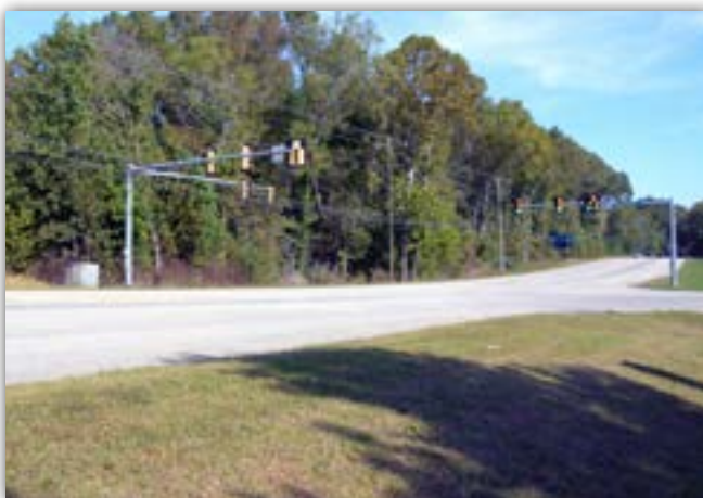
Future location for new roadway at Greenmount Parkway intersection
